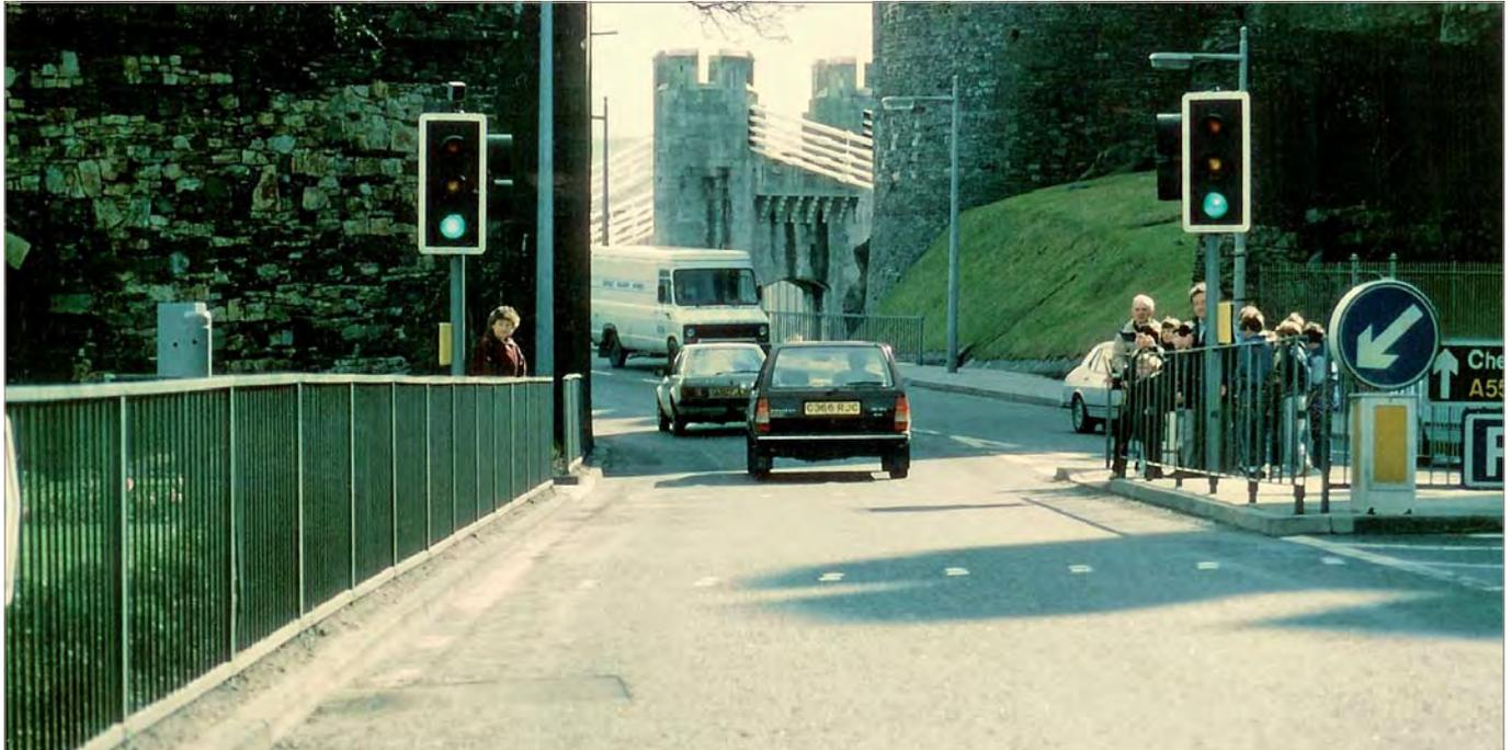
Fig. 1. Children are much safer at guardrails which do not conceal them (right) compared to the traditional concealing design (left)
