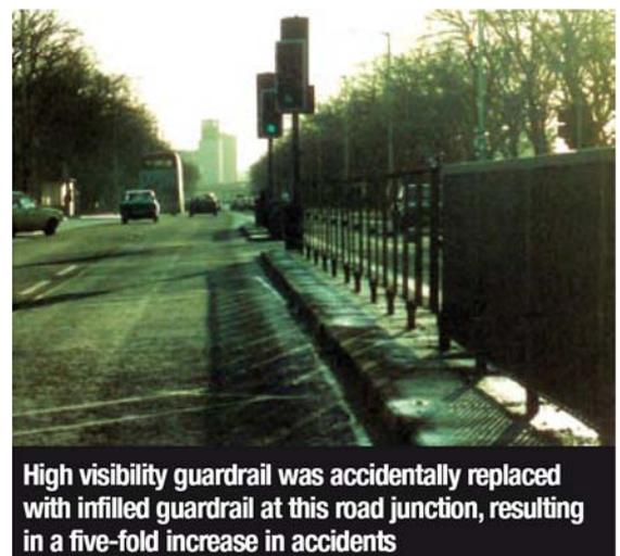
**High visibility guardrail was accidentally replaced with infilled guardrail at this road junction, resulting in a five-fold increase in accidents**
