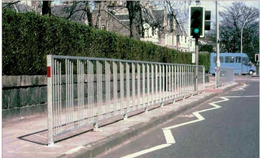
Fig. 4. Optimal use of the new Visiflex guardrail to discourage diagonal crossing and maximise casualty reduction—according to BS 7818,<sup>10</sup> guardrails should extend at least 20 m either side of a crossing
